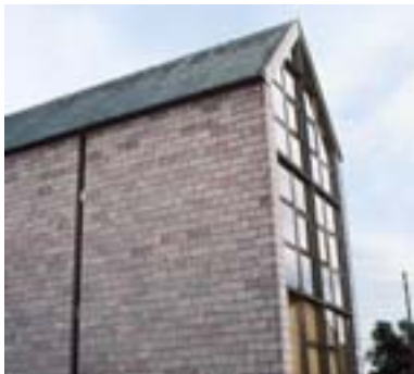
Vodellée - Ing.-arch. J. Delbroek
