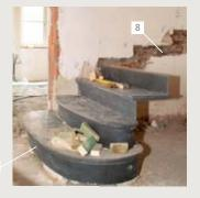
setting facing plaster. As the staircase gradually rises, bricks laid in the plaster come and wedge the step/riser assembly. A distribution vault made of brick comes and solidly fastens the staircase ending in a bottom vault, itself smoothed with plaster. The assembling of the bricks is designed in such a way that the overall assembly is self-supporting. The assembling of the steps and risers therefore determines the vault and not the opposite.
