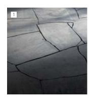
2 An irregular pattern is made from originally rectangular blue limestone flags. The largest offcuts are laid on the circumference and in the middle of the space to be paved. The remaining space is filled with smaller pieces. Random bond requires meticulous workmanship on site if the overall aesthetic harmony is to be achieved.
