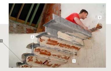
The characteristic feature of this construction method is that there is no template and shuttering. The anchor shoe made of hollow bricks is placed first. The risers and steps are laid alternatively one on the other, simply secured in a 5 cm groove made in the wall and plastered from behind using a fast-
