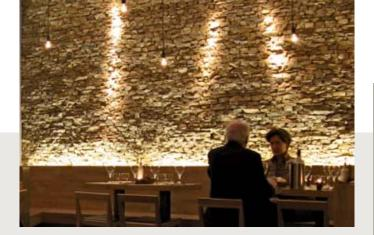
The bonding of this internal dividing wall is an assembly of stones adjusted on the spot and the actual stones are laid on steel angle irons, placed horizontally every metre. The stone fragments are firstly fixed by adhesive cement and invisibly pointed by adhesive less than 2 mm thick.
