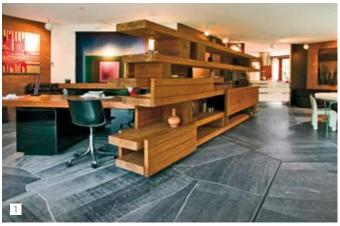
1 Here, the onsite cutting work was raised to a maximum with very fine joints. The cutting line is precise. The final rendering is fairly sophisticated: the advantage of this paved floor is the result of the very clear-cut dimensions between large and small stones, which lightens the overall perception.
