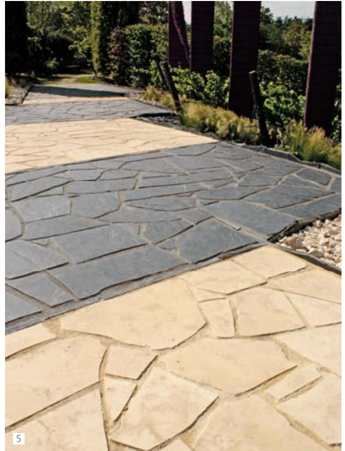
5 COLOURED JOINTS: The joints add the finishing touch to a paved area! Thin or thicker joints, the decision depends on whether you wish to create a traditional, contemporary or natural atmosphere. The colour is also a crucial point and it is worth giving it a lot of consideration before laying the stones. In this theme park where originality was a welcome feature, random bond or opus incertum provides an alternating pattern of shale and white stone. The joints harmonise with the stone for a strikingly graphic result. TERRA BOTANICA, ANGERS (F), DESIGNED BY THIERRY HUAU
