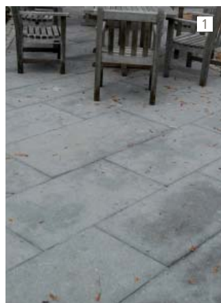
1 Vinalmont limestone is a Meuse limestone lighter than blue limestone. It's elegant and has a very fine grain. PRIVATE GARDEN, LUXEMBOURG (L), DESIGN BY WIRTZ INTERNATIONAL S.A.
