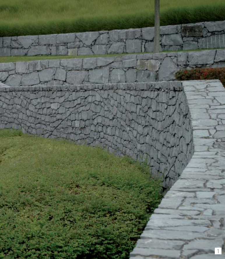
1 A bonding similar to that of the Diegem walls was used again in Luxembourg. They are coupled with walls using very large and very small-sized blocks. The perception of each type of wall is interesting, but the interest also stems from the confrontation of the different bonding within the same perspective.
