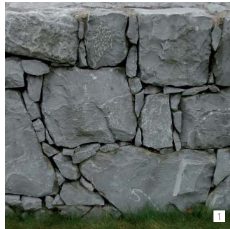
1 A bonding similar to that of the Diegem walls was used again in Luxembourg. They are coupled with walls using very large and very small-sized blocks. The perception of each type of wall is interesting, but the interest also stems from the confrontation of the different bonding within the same perspective.
