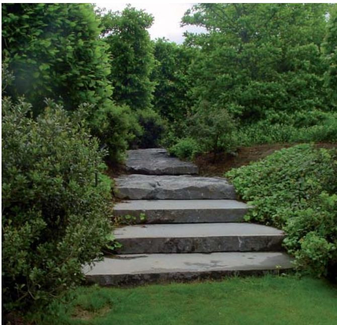
3 The stairway shown here starts with sawn blue limestone with blue limestone crusts taking over halfway up to mark a change in style between two adjoining areas.
