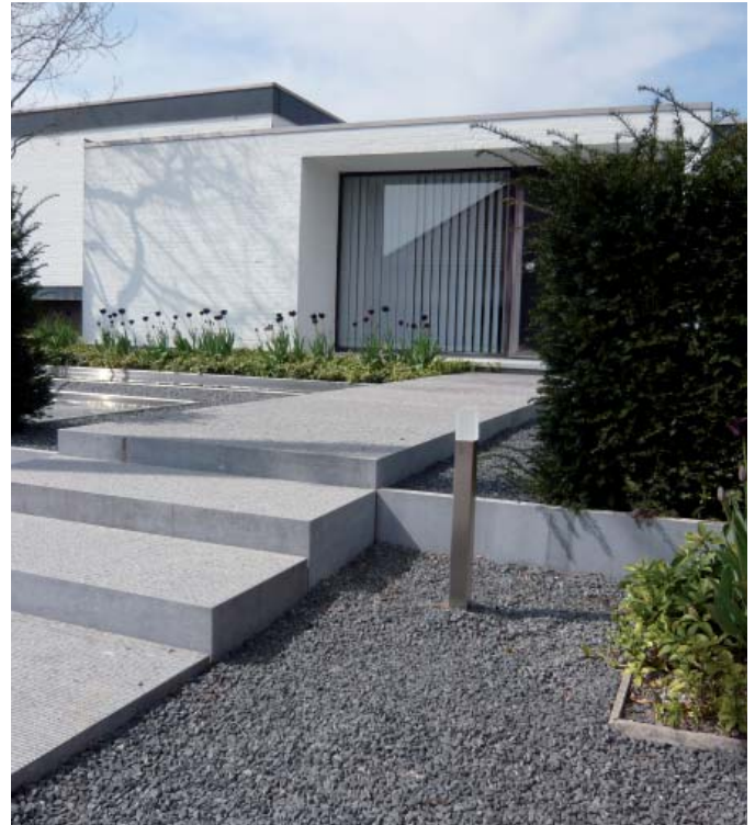
4 One way of producing a stairway with only a few steps is to install the blocks vertically. In this case, the joints have to be made using a water-resistant mortar.
