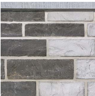
Split and sand-blasted rubble stones
