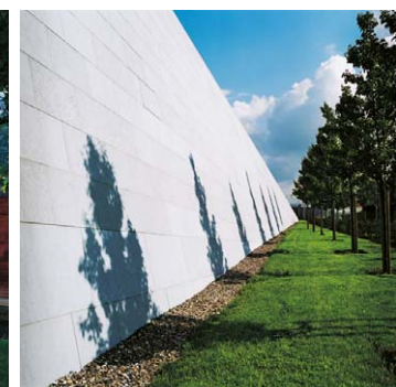
Liège, Val Benoît bridge, planning office R. Greisch, 1997-2000
