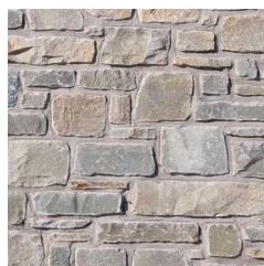
Roughly cleaved rubble stone masonry
