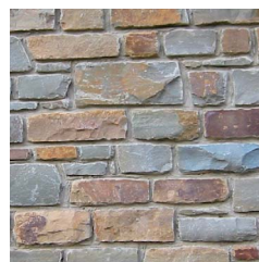
Semi-dressed rubble stone masonry
