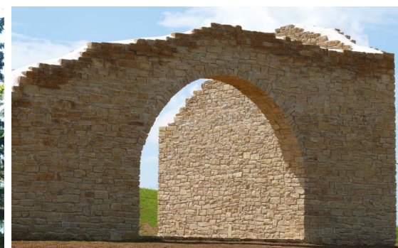
Dry stone masonry
