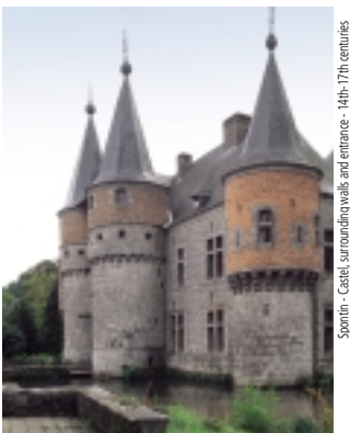
Spothin - Caesl, surrounding wall and entrance - 14th-17th centuries
