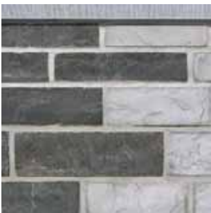
Split and sand-blasted rubble stones
