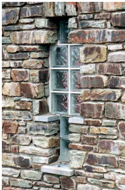
Florenville, light socket in a garage, arch. R. Debrémaison
