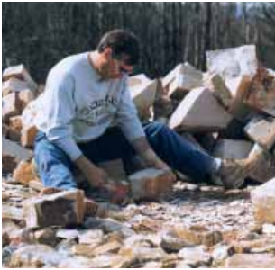
Hammering rubble stone
