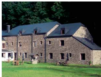
Lafoët, Hotel "Le moulin Simonis"
